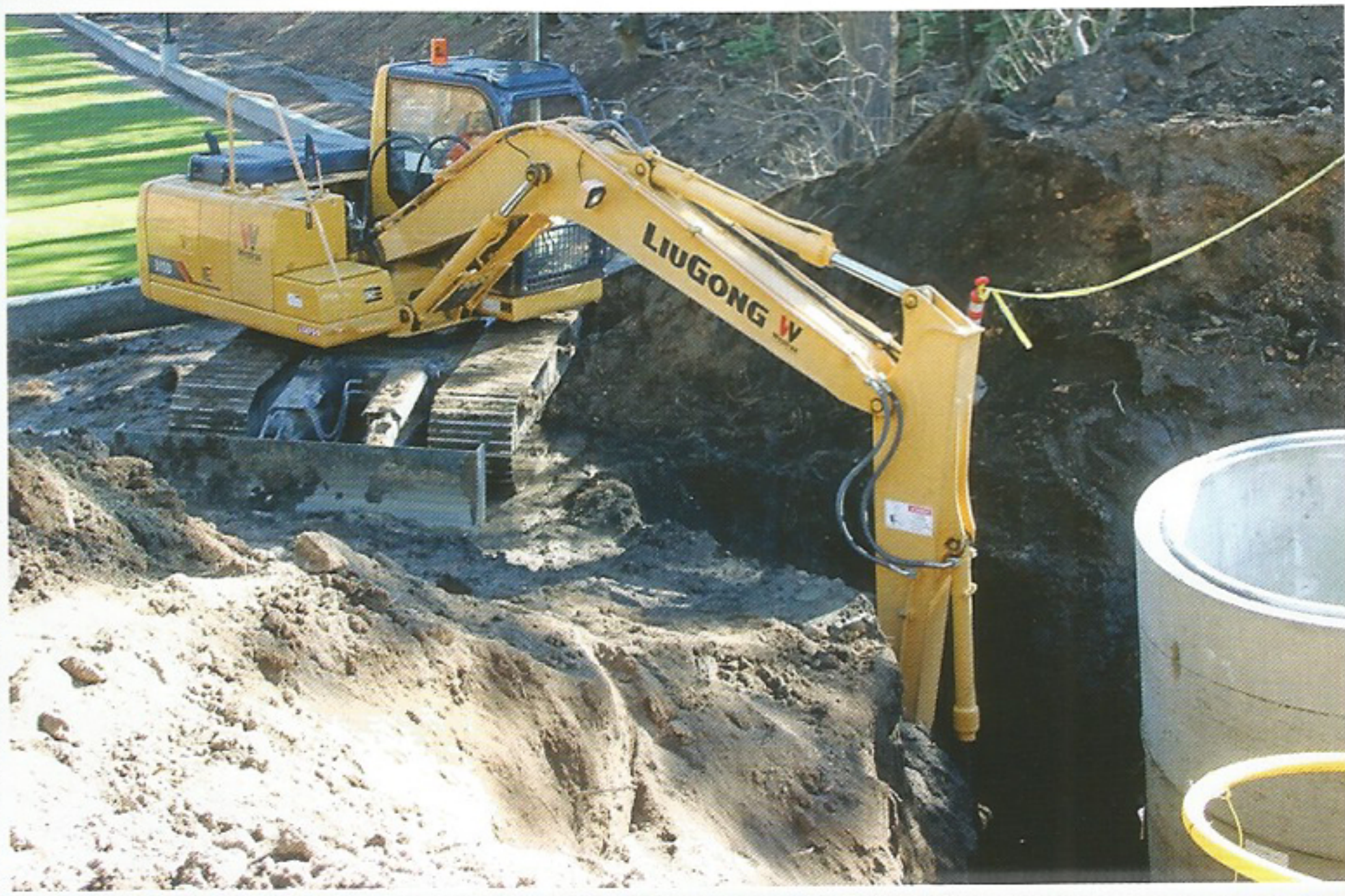
Above Left: Trenching for lift station.
